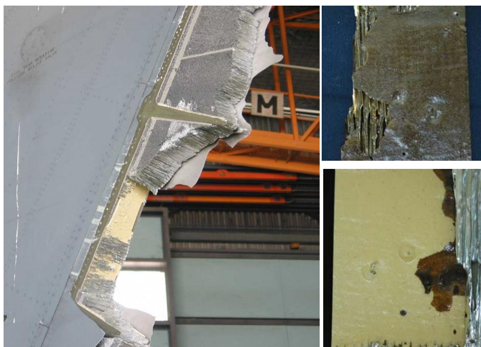
Figure 23. An injection repair to an aircraft rudder that failed in flight.
